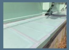
Waterproofing of the bases of anchor bolt shafts and tops of boxes around outdoor tanks
