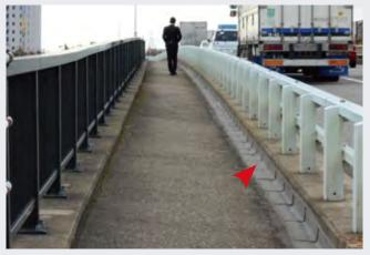
The system accommodates the differential movement of the carriageway and the pedestrian bridge maintaining a weatherproof seal and preventing water leaks.
