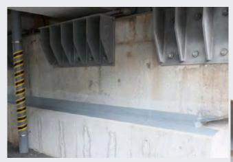
Waterproofing between the old column and the new concrete jacketing prevents rainwater penetration into the joint of the concrete jacketing. Long-term seismic resistance can be expected.
