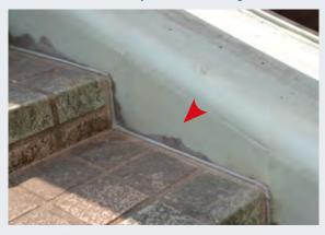
Catpad-Cloth was applied to the side wall of these steps. It prevented the formation of rust and prevented water from being trapped or stagnating from the flow of rainwater from the upper stages.
