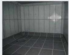
Sheet edges are covered and sealed with Cat-Tape Clear.
