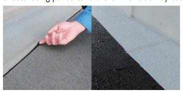
If this occurs, the outermost edges should be left unsealed. Catpad accommodates movement in a sideways direction.
